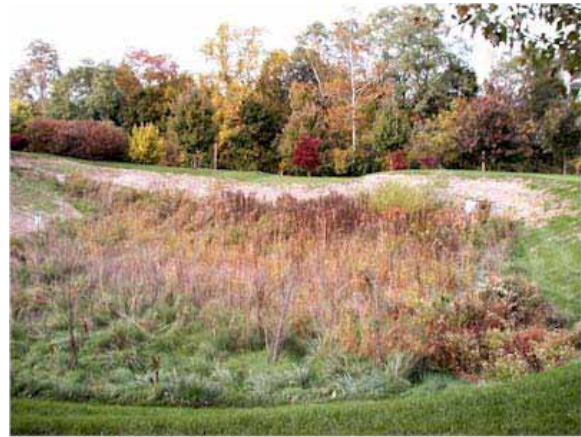
FIGURE 5-43 Dry extended detention pond. SOURCE: PaDEP (2006).
