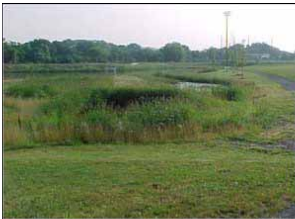
FIGURE 5-40 Constructed wetland at SOURCE: PaDEP (2006).
