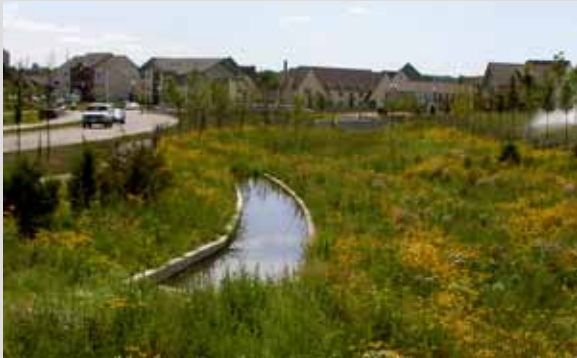
FIGURE 5-57 View of a sediment trap and porous landscape detention area in the central parkway spine of Heritage Park. The sediment trap in the center left of the photo was designed for ease of maintenance access by city crews with standard city maintenance equipment. Courtesy of SRF Consulting Group, Inc.
