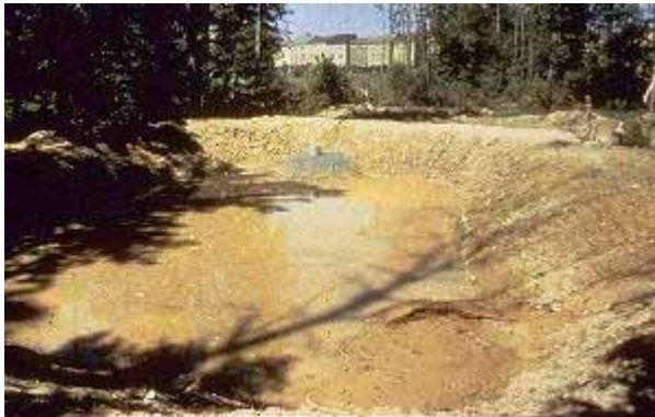
FIGURE 5-8 Sediment filter left in place after construction. SOURCE: Robert Traver.
