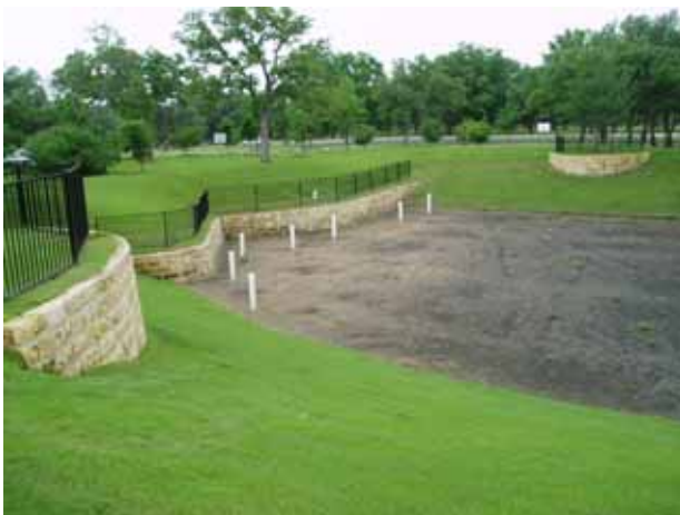
FIGURE 5-45 Austin sand filter. SOURCE: Robert Traver.
