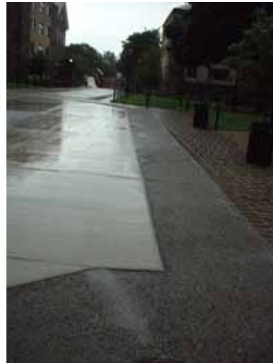
FIGURE 5-31 Pervious concrete at Villanova University. SOURCE: Reprinted, with permission from VUSP. Copyright by VUSP.
