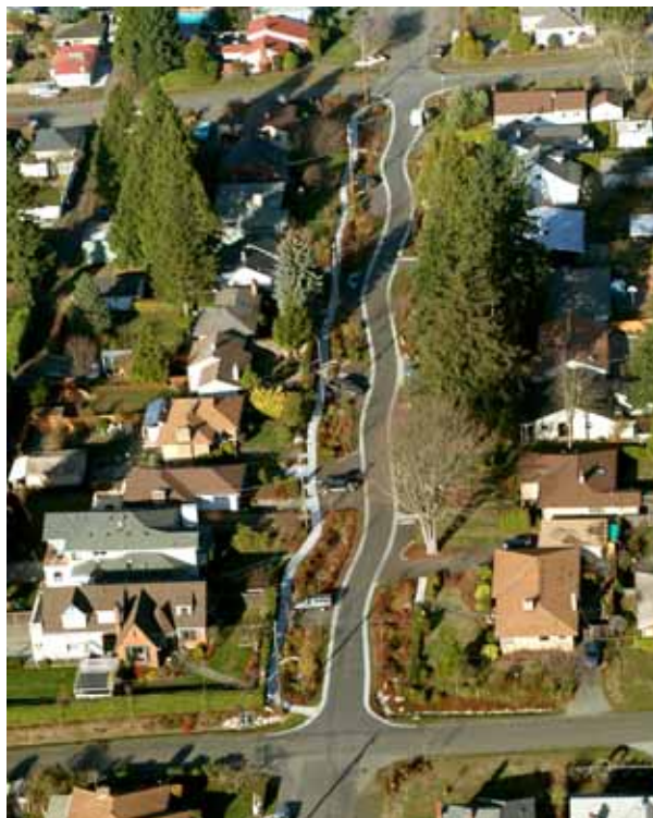
FIGURE 5-6 110 th Street, Seattle, part of the Natural Drainage Systems Project. This location exhibits several elements of impervious cover reduction. In particular, vegetated swales were installed and curbs and gutters removed. There are sidewalks on only one side of the street, and they are separated from the road by the swales. The residences' rooftops have been disconnected from the storm-drain systems and are redirected into the swales. SOURCE: Seattle Public Utilities.
