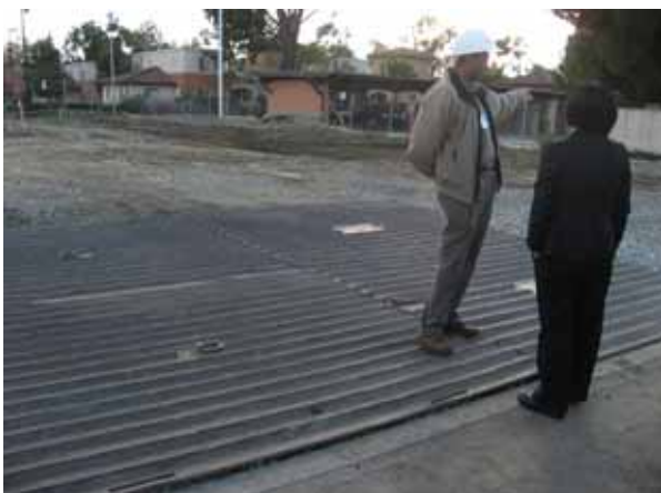
FIGURE 5-10 Rumble strips to remove dirt from vehicle tires. SOURCE: Laura Ehlers.
