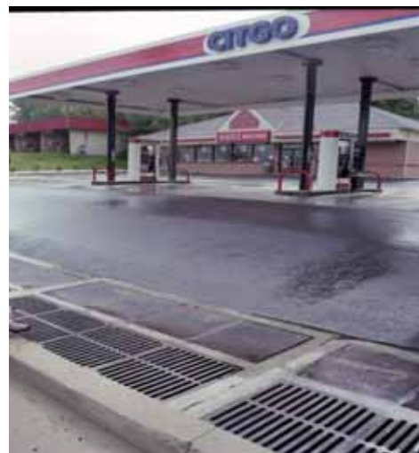
FIGURE 5-46 Delaware sand filter. SOURCE: Tom Schueler.
