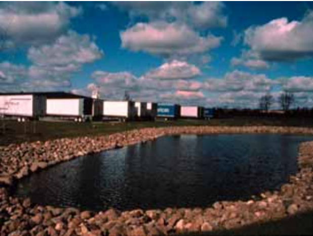
FIGURE 5-3 On-site detention. SOURCE: Tom Schueler.
