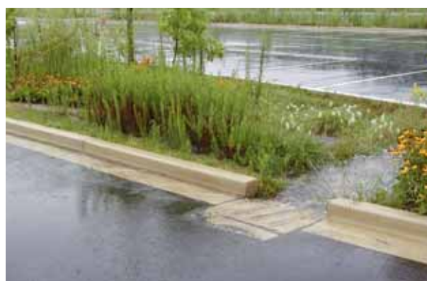
FIGURE 5-17 Bioretention during a storm event at the University of Maryland. SOURCE: Reprinted, with permission, from Davis et al. (2008). Copyright 2008 by the American Society of Civil Engineers.
