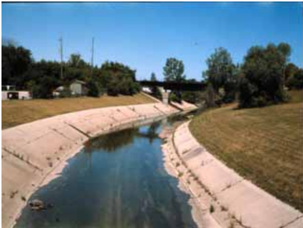
FIGURE 5-2 Concrete channel in Lincoln Creek, Milwaukee, Wisconsin. SOURCE: Roger Bannerman.
