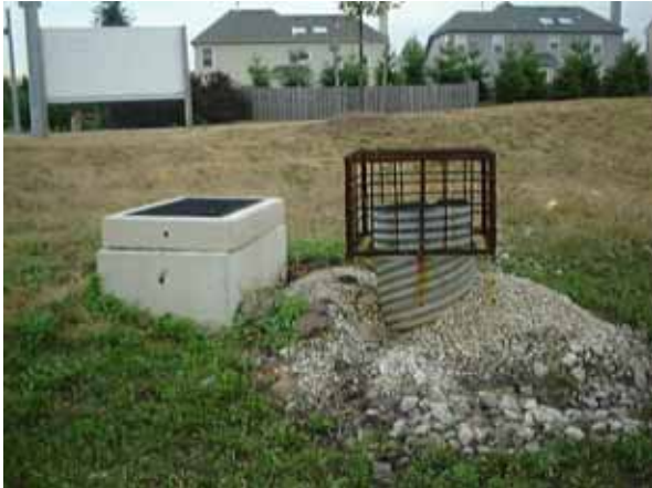
FIGURE 5-8 Sediment filter left in place after construction. SOURCE: Robert Traver.
